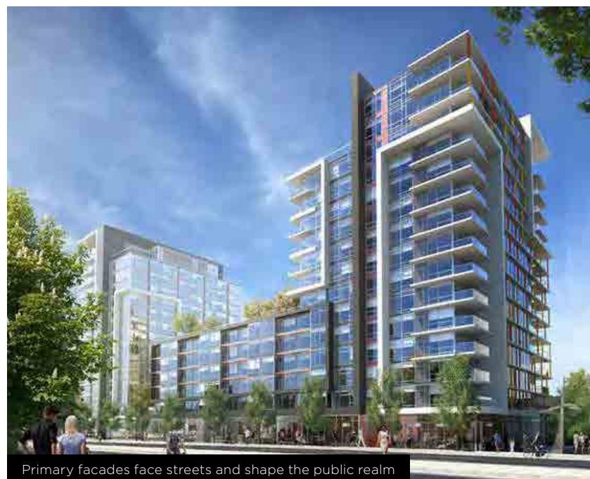
Primary facades face streets and shape the public realm
